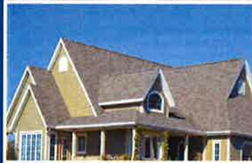
ROOF & WINDOW REPLACEMENT
